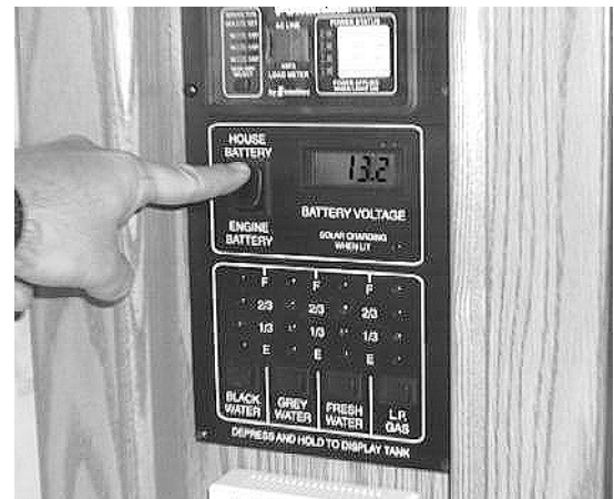
Battery Voltage Check One Place Panel
