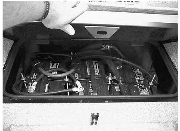
Lift step to access batteries
