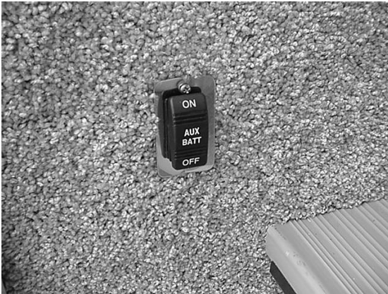
Aux. Batt. Disconnect Switch in Entrance Stepwell
