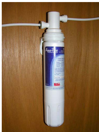
Water Filter Assembly (Located below galley sink)
