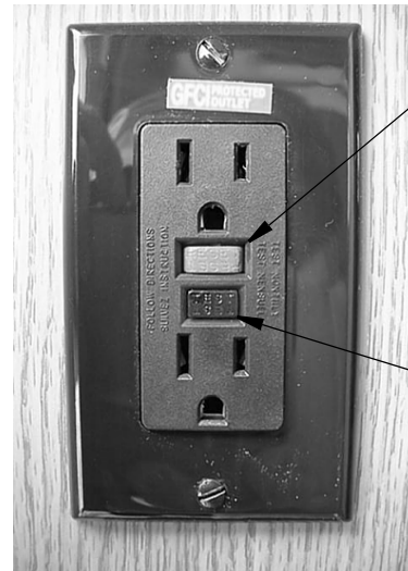
GFCI Outlet (Ground Fault Protector)
