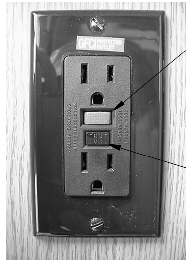
GFCI Outlet (Ground Fault Protector)
