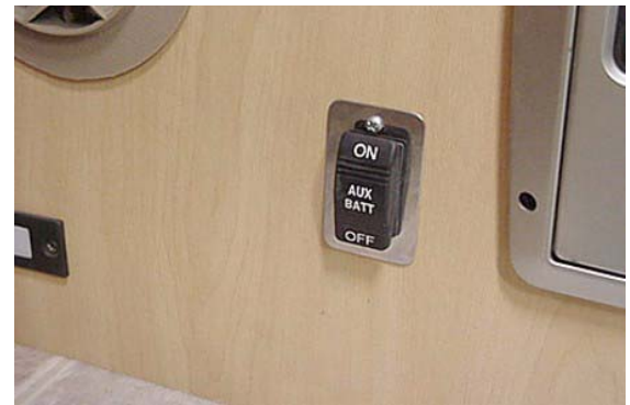
Aux. Batt. Switch - typical (Near entrance door)
