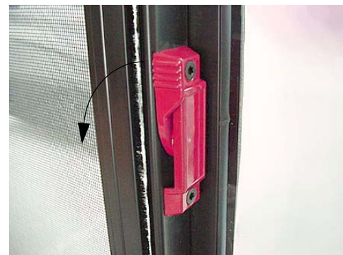
Pull latch outward to slide window open
