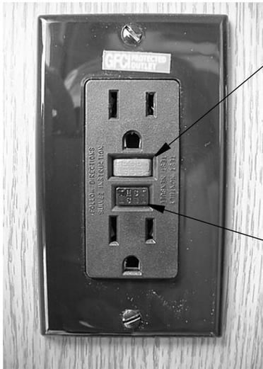
Push to Reset circuit after monthly testing or ground fault tripping.
