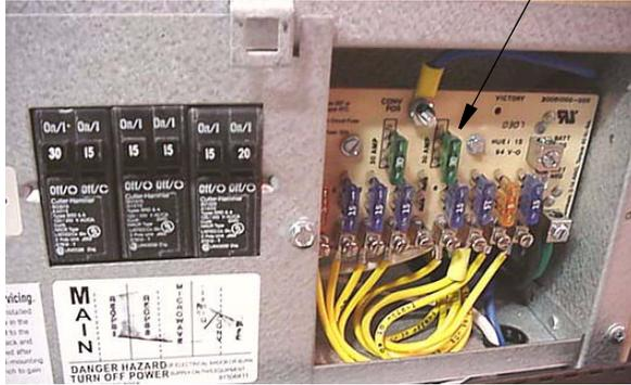
The fuse panel accepts only blade type plug-in fuses. Always replace fuses with those of the same amperage rating.
