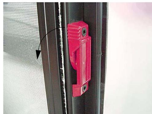
Pull latch outward to slide window open
