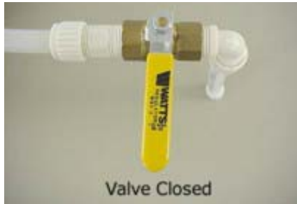
Water Tank Drain Valve (Typical) Under Rear Bed or Couch
