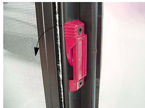
Pull latch outward to slide window open
