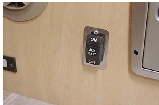
Aux. Batt. Switch - typical (Near entrance door)
