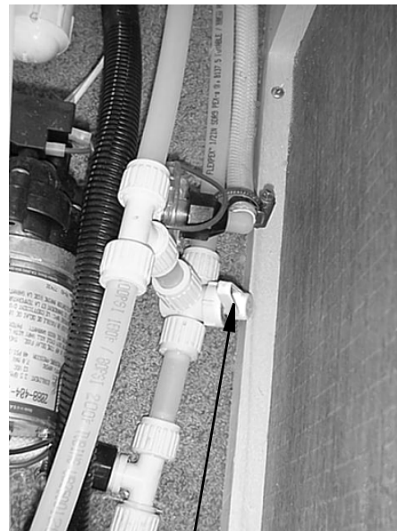
Waterline Drain Valve (Typical)
