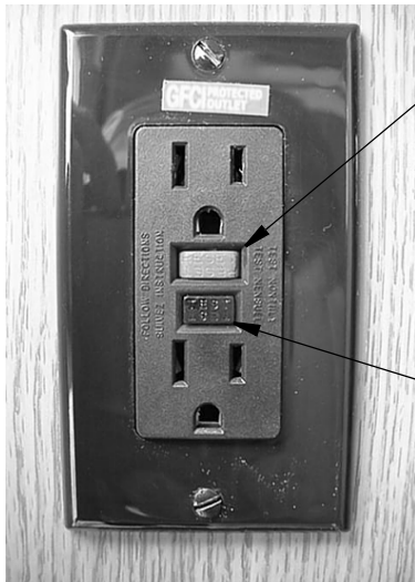
GFCI Outlet (Ground Fault Protector)
