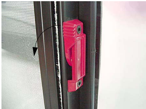
Pull latch outward to slide window open
