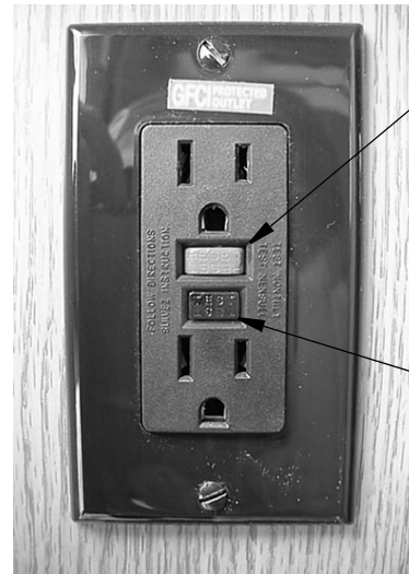
GFCI Outlet (Ground Fault Protector)
