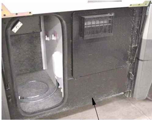
Water Pump Access Panel (Typical)
