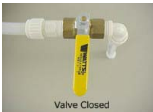
Water Tank Drain Valve (Typical)
