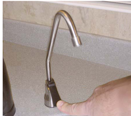
Filtered Water Faucet -Typical View
