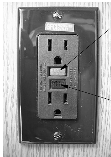
GFCI Outlet (Ground Fault Protector)
