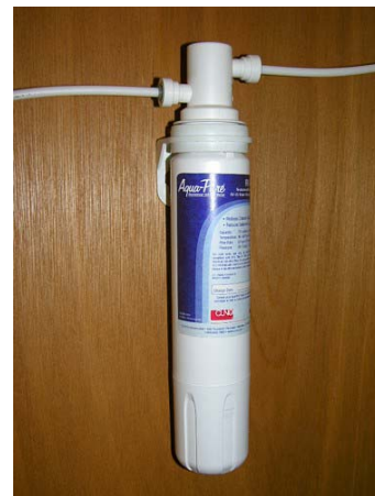
Water Filter Assembly (Located below galley sink) -Typical View
