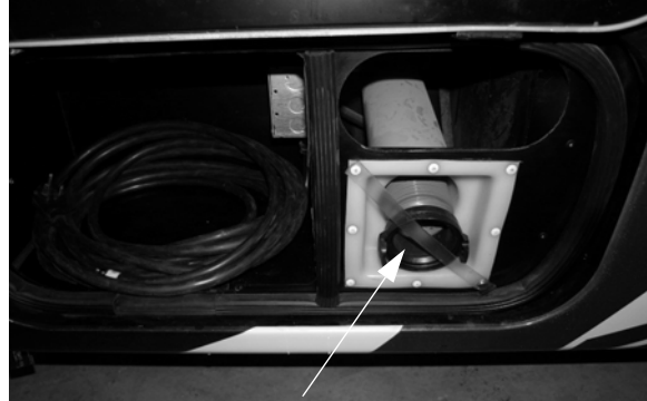
Sewage Drain Hose (Located in utility compartment)
