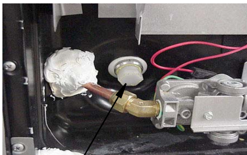
Water Heater Drain Plug (Remove with socket)
