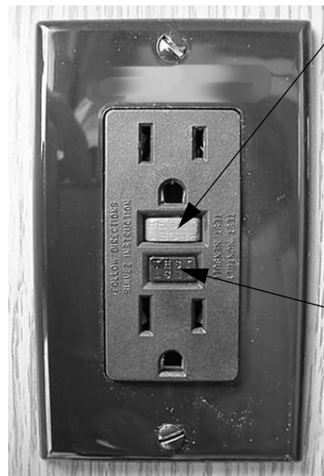
GFCI Outlet (Ground Fault Protector)
