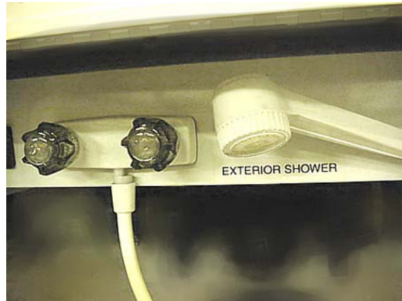
Exterior Shower/Wash Station -Typical View
