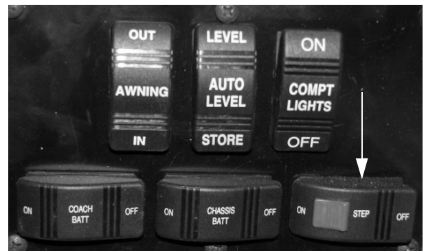
Entry Step Switch (Located near the entrance door) -Typical View
