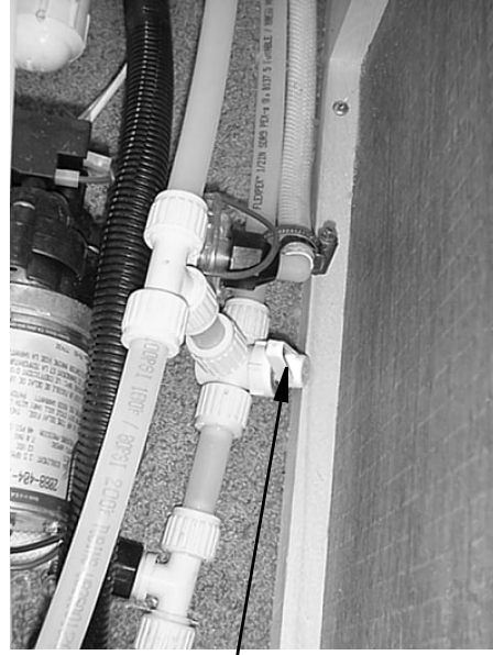
Waterline Drain Valve (Typical)
