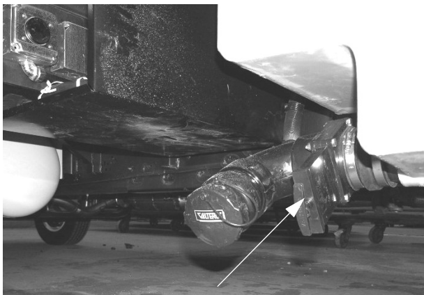
Black Waste Tank Drain Valve (Located beneath coach on mid-driver side) -Typical View
