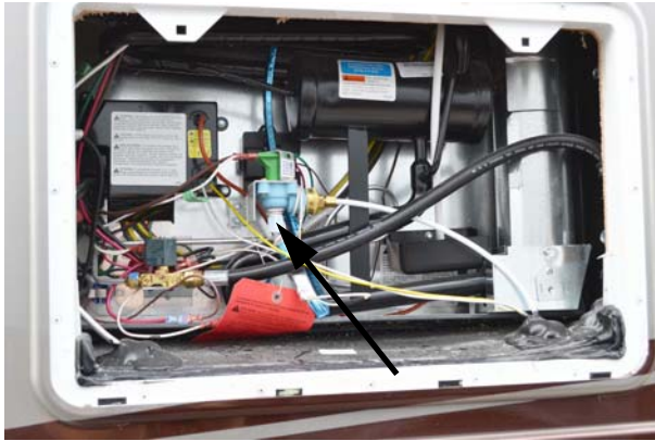
Ice Maker Water Supply Connection -Typical View
