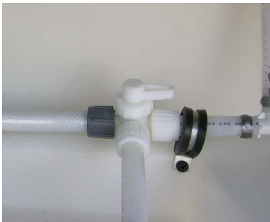
Waterline Drain Valve -Typical installation shown
