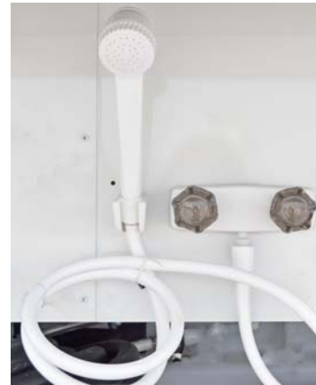
Exterior Shower/Wash Station -Typical View
