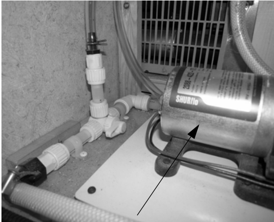
Water Pump -Typical installation shown
