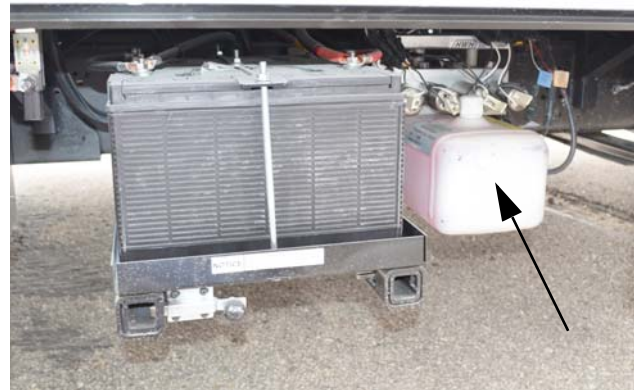
Hydraulic Oil Reservoir (Located in mid-passenger side compartment) -Typical View
