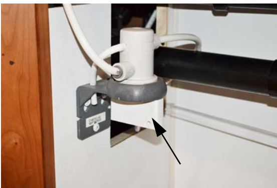
Diverter Plug (installed in filter socket)
