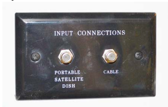
Cable TV/Satellite Dish Connections (Located in backwall compartment) -Typical installation shown
