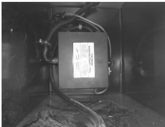
Automatic Power Transfer Box (Located inside utility compartment) -Typical installation shown
