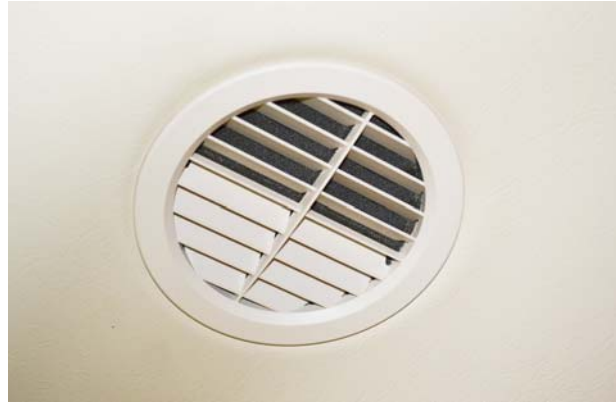
Return Air Vent (Shown with filter installed) -Typical View
