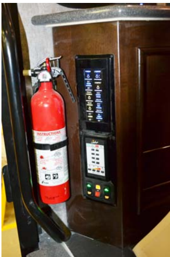
Fire Extinguisher (Located near entrance door) -Typical installation shown
