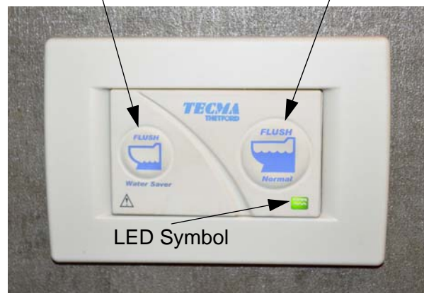
Wall Switch/Controller (Located on wall near toilet)
