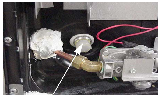
Water Heater Drain Plug (Remove with socket)
