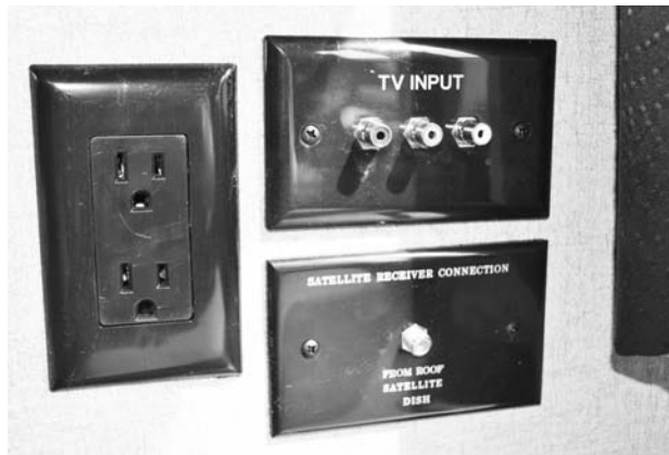
Bedroom DVD/Satellite Receiver Connection -Typical View
