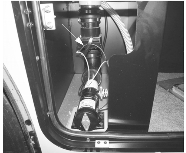
Black Waste Tank Drain Valve #1 (Front) (Located in passenger side compartment ahead of rear axle) -Typical View
