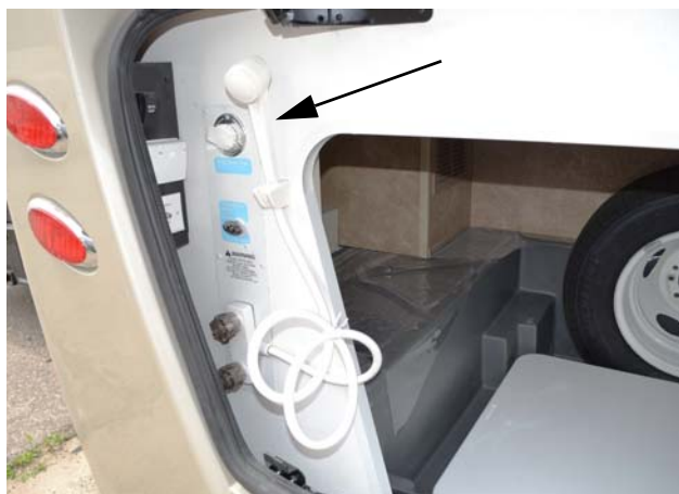
Exterior Shower/Wash Station (Located in backwall exterior service center)
