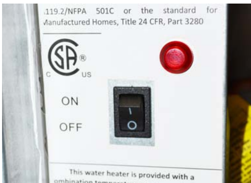
Water Heater (Tankless) Power Switch -If Equipped
