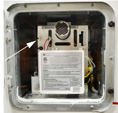
Water Heater Power Switch (Located inside water heater door) -If Equipped
