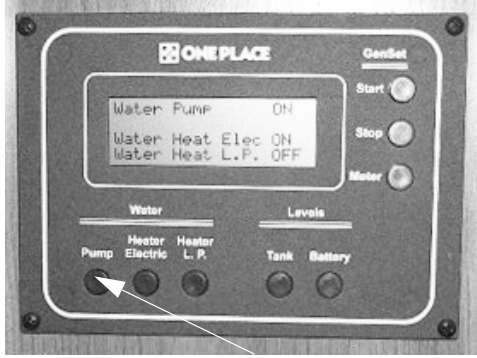
Water Pump Switch
