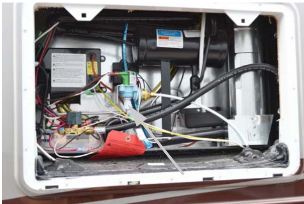
Ice Maker Water Supply Connection -Typical View
