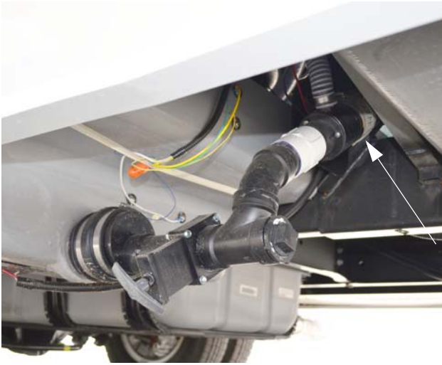
Waste Pump (Located on driver side of coach behind rear wheel) -Typical View
