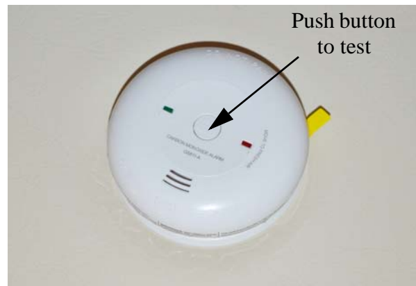
Carbon Monoxide Alarm (9V Battery Required) - Press the Test/Reset button weekly to test
