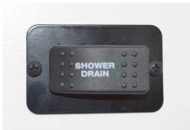
Shower Drain Switch (Located near shower head) -Typical View
