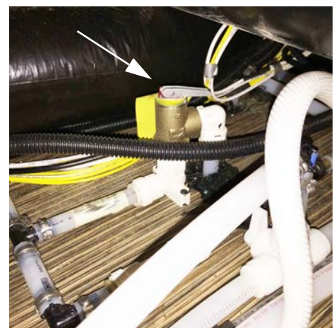
Pressure Temperature Relief Valve (Lift handle only when water heater is cold)
