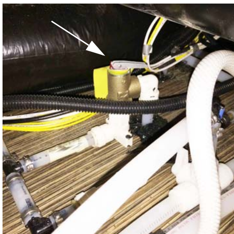
Pressure Temperature Relief Valve (Lift handle only when water heater is cold)
