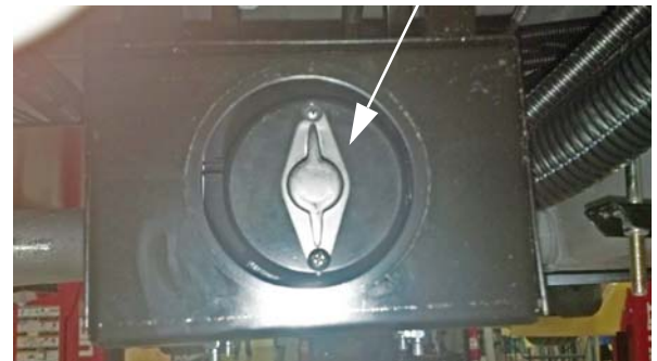
Waste Pump (Located beneath coach)
