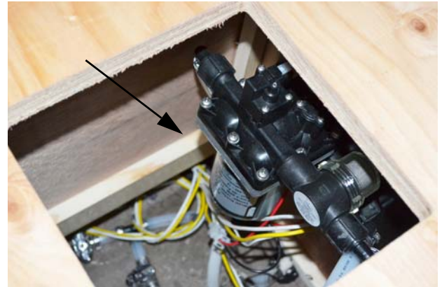
Water Pump (Located beneath bed) -Typical installation shown
