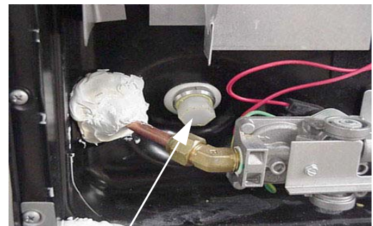
Water Heater Drain Plug (Remove with socket)
