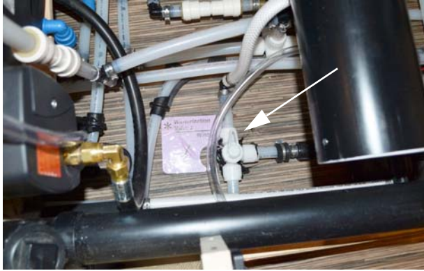
Winterization Valve 2 (See “Water System Drain Valve Locations” chart at the end of this section for location on your model)
