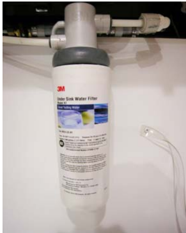
Cold Water Filter Assembly (Located inside lower galley cabinet) NOTE: Hot waterline is not filtered.
