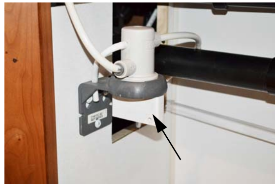
Diverter Plug (installed in filter socket)
