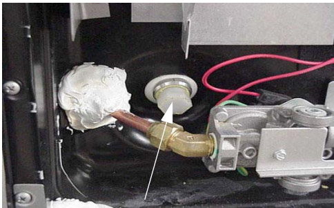
Water Heater Drain Plug (Remove with socket)
