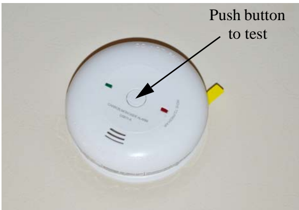
Carbon Monoxide Alarm
