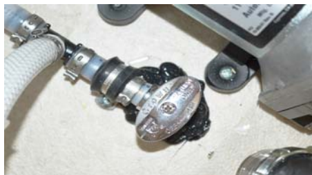
Drain Valve (Typical)
