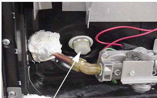
Water Heater Drain Plug (Remove with socket)
