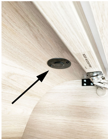
Roof Access Port -Typical View
