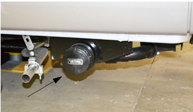
Sewage Drain Outlet (Located beneath motorhome) *Model 59K
