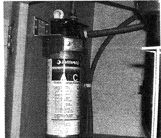
Water Filter Assembly - Below Galley Sink
