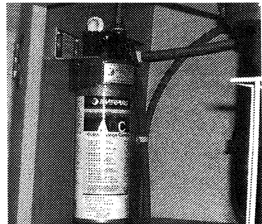
Water Filter Assembly - Below Galley Sink
