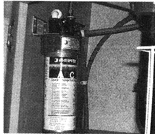
Water Filter Assembly - Below Galley Sink
