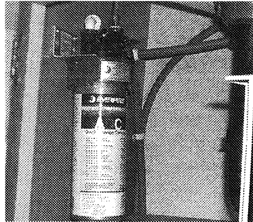
Water Filter Assembly - Below Galley Sink
