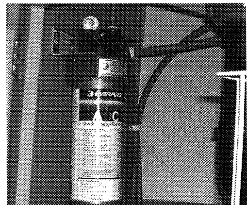
Water Filter Assembly - Below Galley Sink
