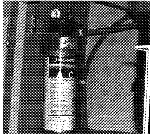
Water Filter Assembly - Below Galley Sink
