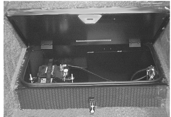
House Battery in Top Entrance Step
