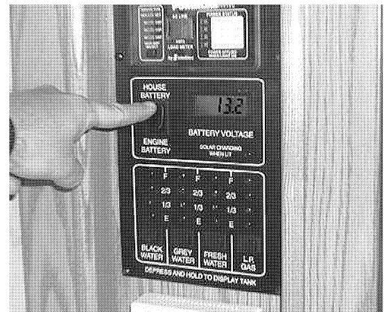
Battery Voltage Check One Place Panel
