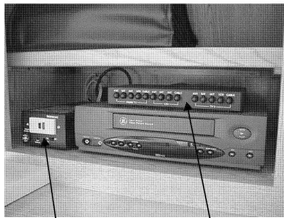
DC/AC Inverter Video Selector System
