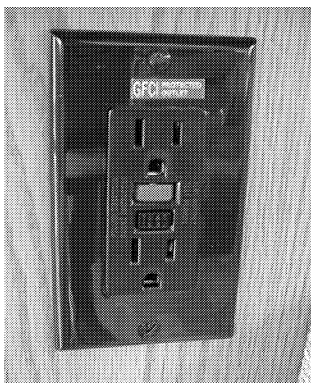
GFCI Outlet (Ground Fault Protector)
