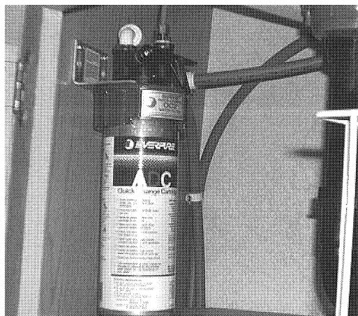
Water Filter Assembly - Below Galley Sink
