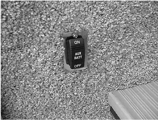
Aux. Batt. Disconnect Switch in Entrance Stepwell
