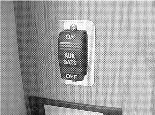
Aux. Batt. Switch (Near entrance door)
