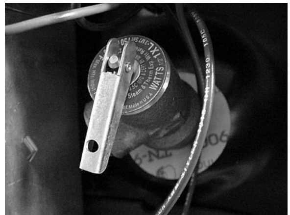
Lift straight out to open P-T valve
