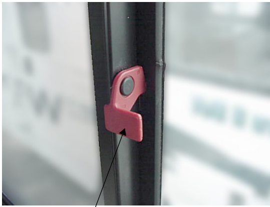
Lift Latch to Open Window (Be sure handle is also raised when closing)
