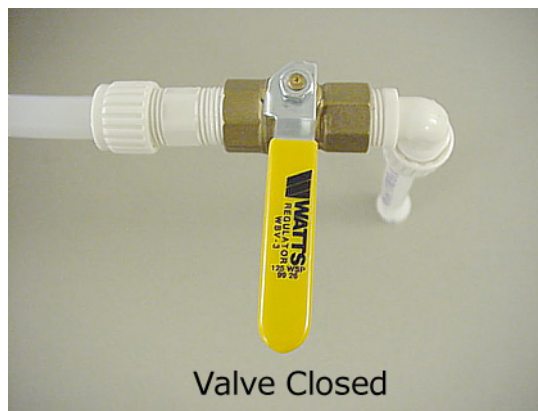
Water Tank Drain Closed
