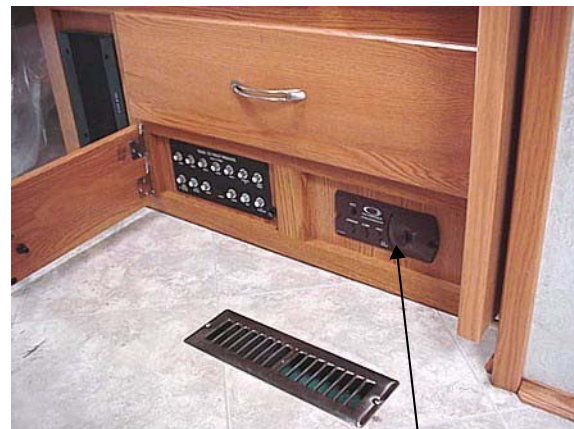
LP Gas Alarm
