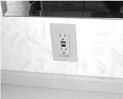
Ground Fault Circuit Interrupter (GFCI)
