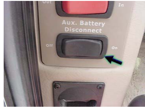
Aux. Batt. Switch (on entry panel)
