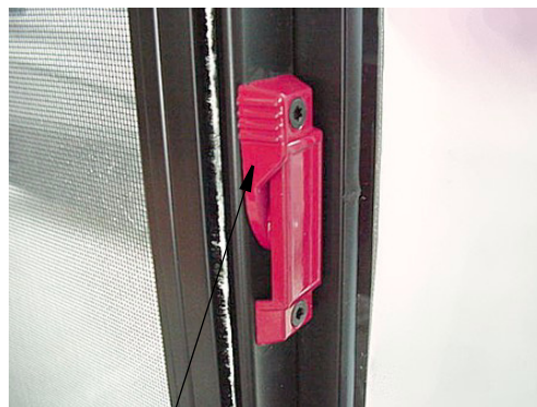
Pull latch outward to slide window open
