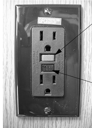
GFCI Outlet (Ground Fault Protector)
