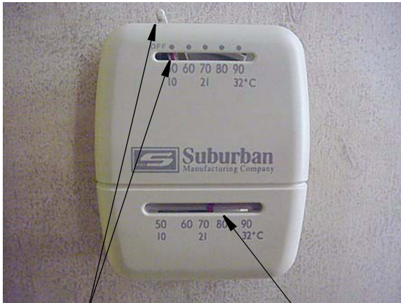
Thermostat/Switch • Move from OFF to desired temperature for furnace operation Room Temperature Thermometer
