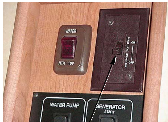
Diesel Engine Heater Switch (typical)
