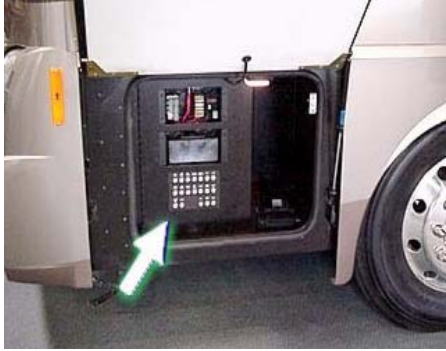
12V Electrical Compart-
