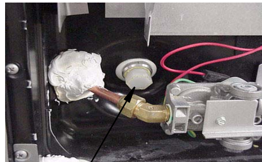
Water Heater Drain Plug (Remove with socket)
