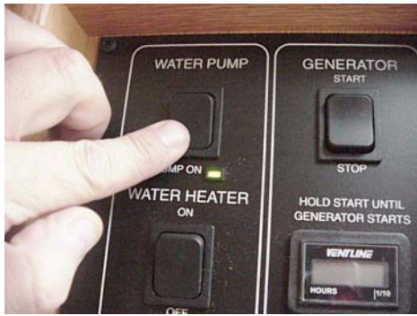
Water Pump Switch (Located on OnePlace® Monitor Panel)
