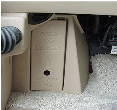
Automotive 12-Volt Circuit Breakers and Fuses (Located beneath left end of dash) -Typical View
