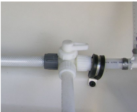
Waterline Drain Valve -Typical installation shown
