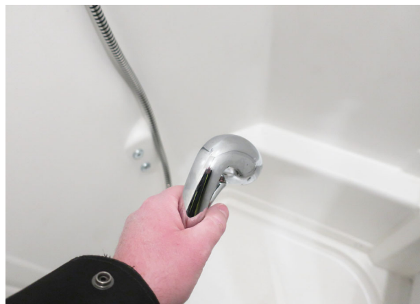
Point shower head at the drain and squeeze until water stops flowing. -Typical View
