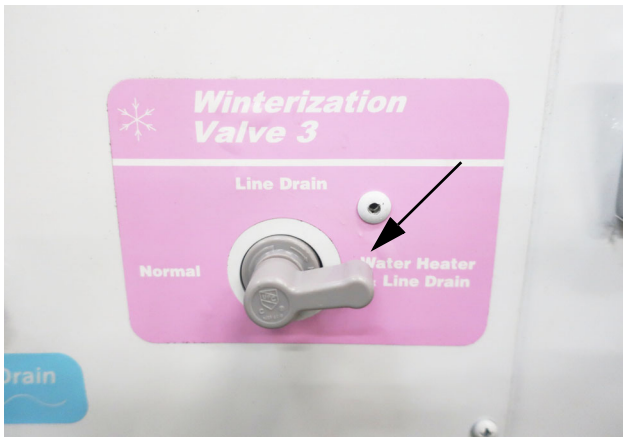
Winterization Valve 3 (Turn it to the Water Heater and Line Drain position). -Typical View
