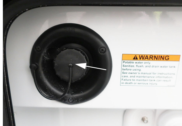
Water Tank Gravity Fill (Located in the water center) -Typical View
